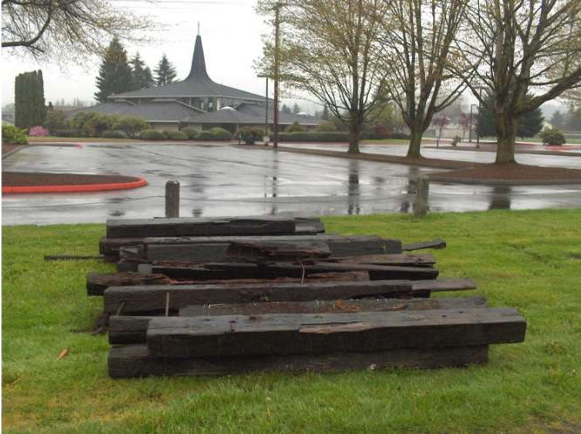
Fix-It Day, May 14, deteriorated ties removed
